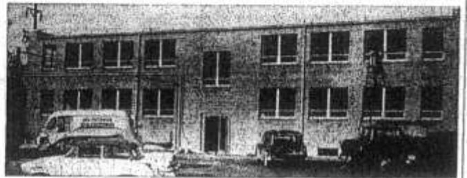
A. J. Elme's new, two-story office building on Shelbyville Road, valued at $75,000 to $100,000 ought to be ready in a few weeks. Finishing work is presently underway.
